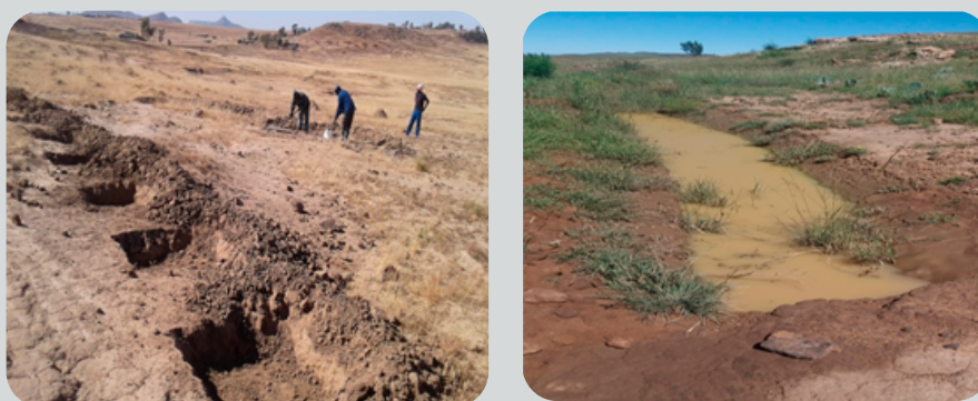
Figure 4.25: Infiltration pits and trenches to promote groundwater recharge and rehabilitate degraded landscapes – Mafeteng district
