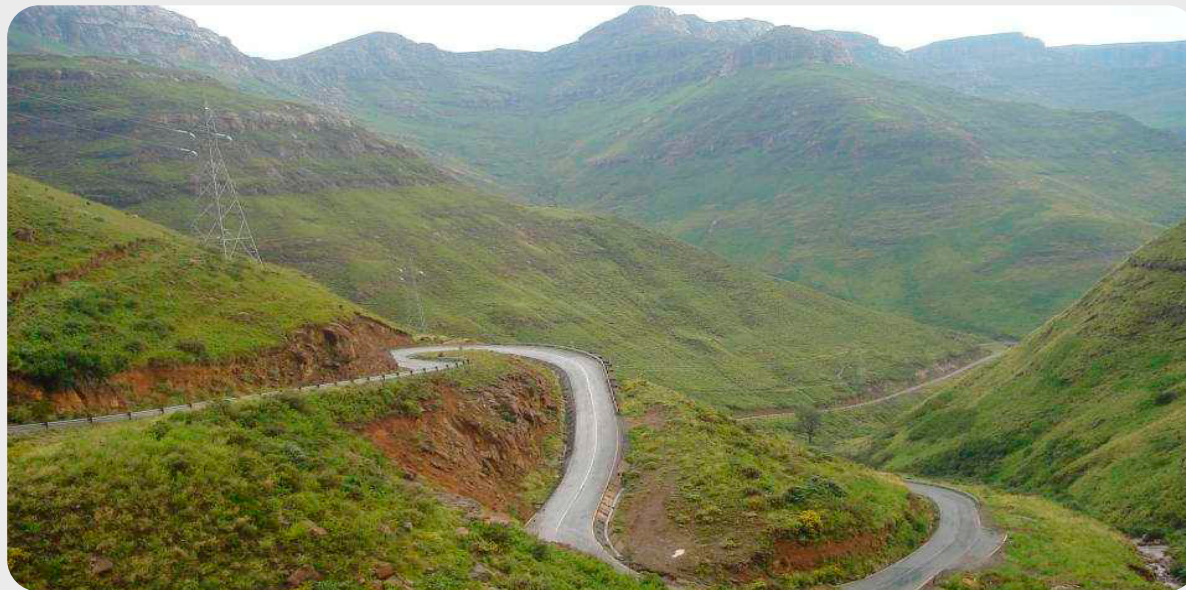
Figure 3.7: Example of common road network in Lesotho (Adriaan Geldenhuys, Egan's Altitude Adventures 2013)
